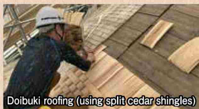
To-in Rai-do after the completion of doibuki roofing
