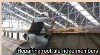
Doibuki roofing (using split cedar shingles)
