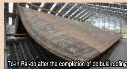
Doibuki roofing (using split cedar shingles)
