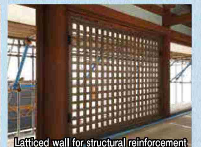
Latticed wall for structural reinforcement
