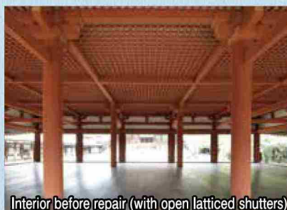
Interior before repair (with open latticed shutters)
