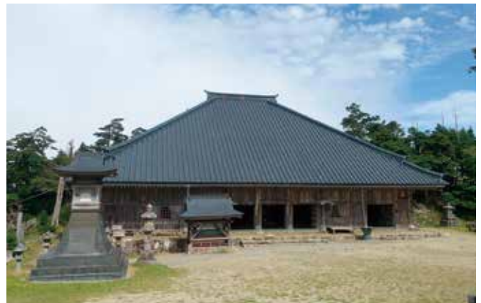
The 67 th gyosho Omimesan-ji Hondo (provided by Omimesan-ji) The Hondo had been built by 905. Two gold Buddha statues were unearthed, amongst other things, during dismantling and repair work.
