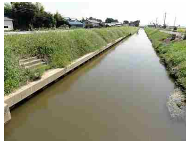
○排水路 (○○市○○町○○地内)
