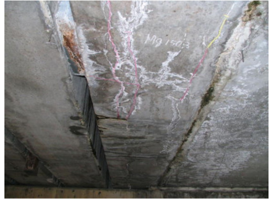
図9 PC桁のひび割れ・遊離石灰
